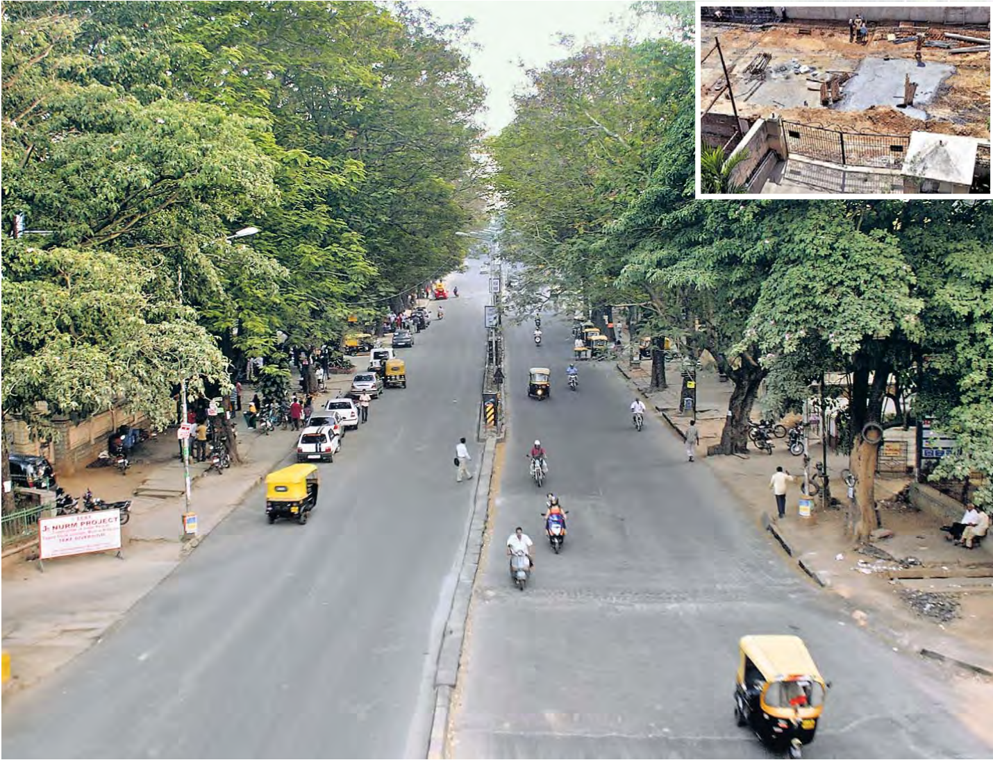
VICIOUS CIRCLE: KR Road, which leads to Tagore Circle (inset) where a controversial underpass is under construction
