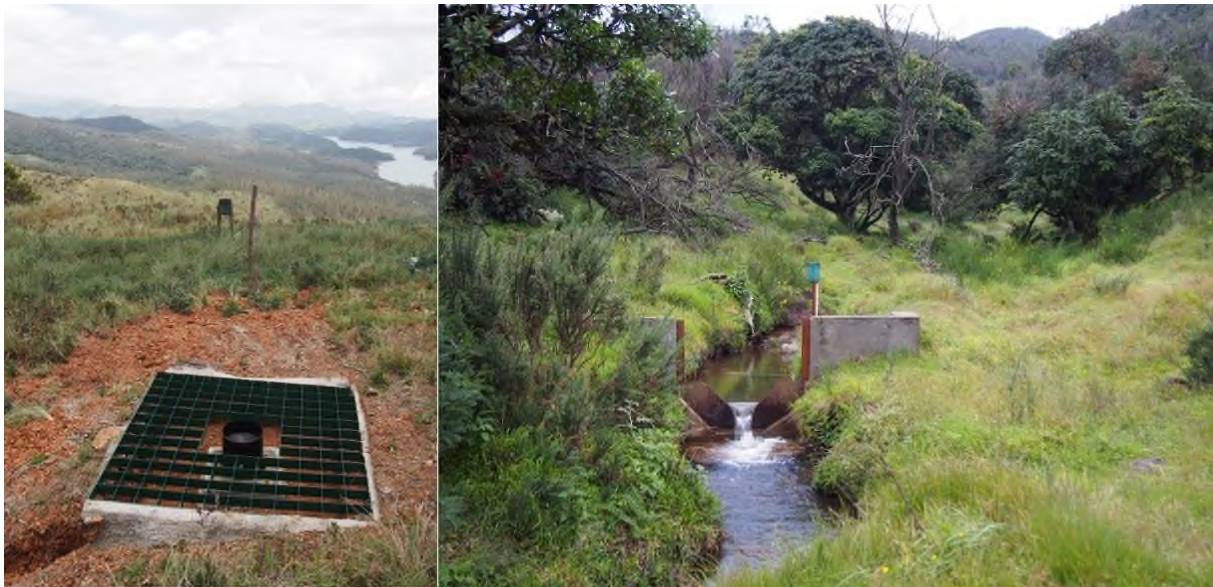
Figure 3-1: An example of a rain gauge installation (left) and headwater stream gauge (right) within our network in the Nilgiris area of the Western Ghats.
