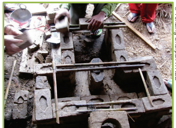
Trainees prepare the frame for an improved cook stove at Rampuria village
