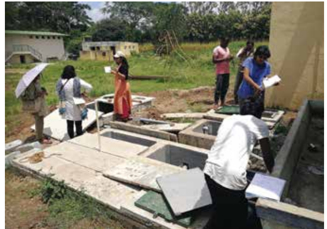
Left: Inspecting the first flush rainwater harvesting. © Lakshmi Raveendran.
